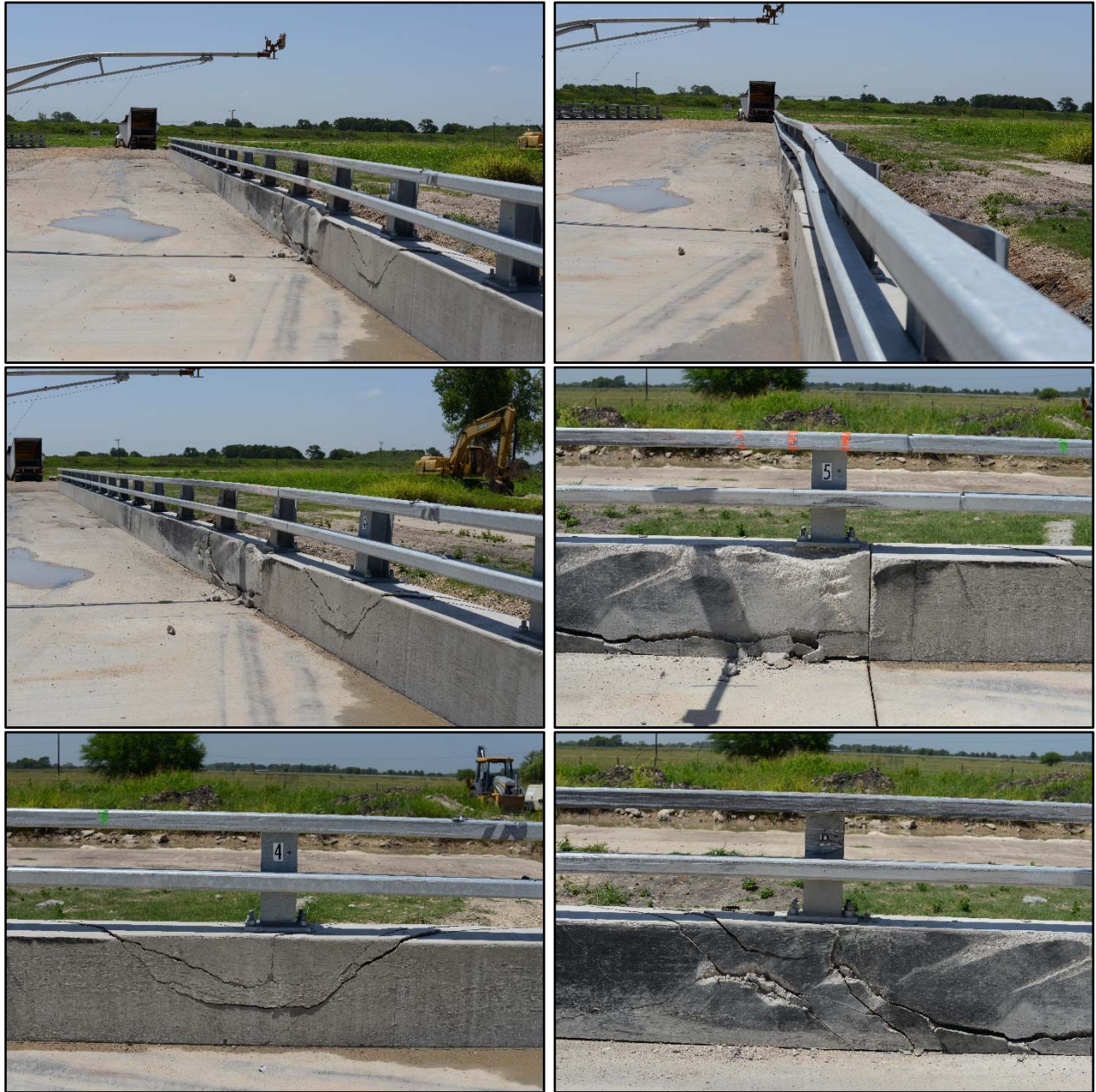
Figure 7.3. PennDOT PA Bridge Barrier after Test No. 609591-03-3.
