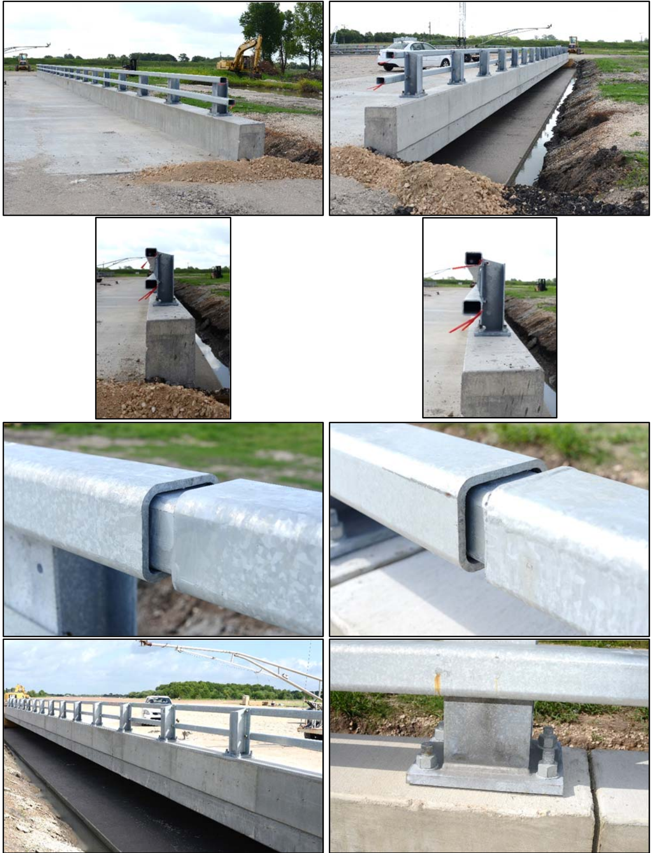
Figure 2.2. PennDOT PA Bridge Barrier prior to Testing.
